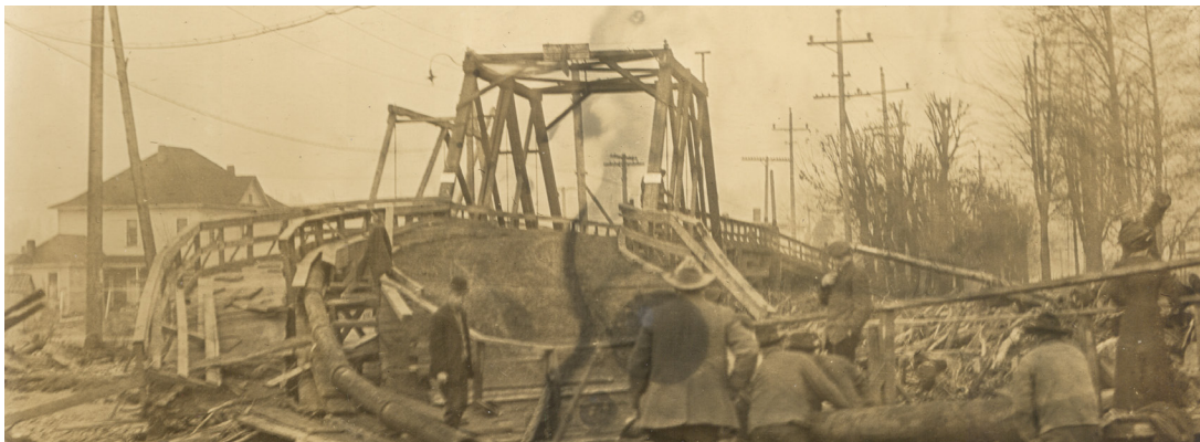
The Flood of 1911 destroyed the County Bridge (Bronson Way Bridge) across to the Sartoris' North Renton properties. (RHM# 2000.054.5374)
